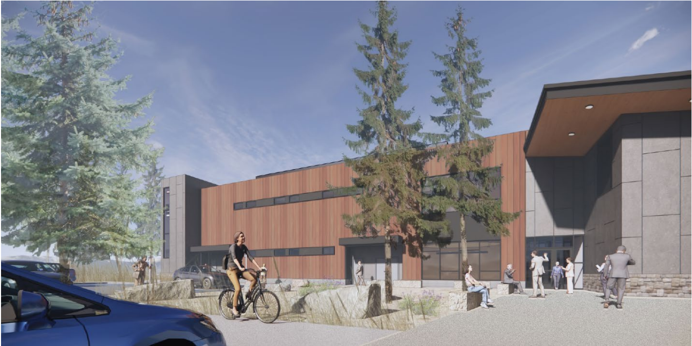
FIGURE 4: NORTH VIEW - STAFF ENTRANCE
