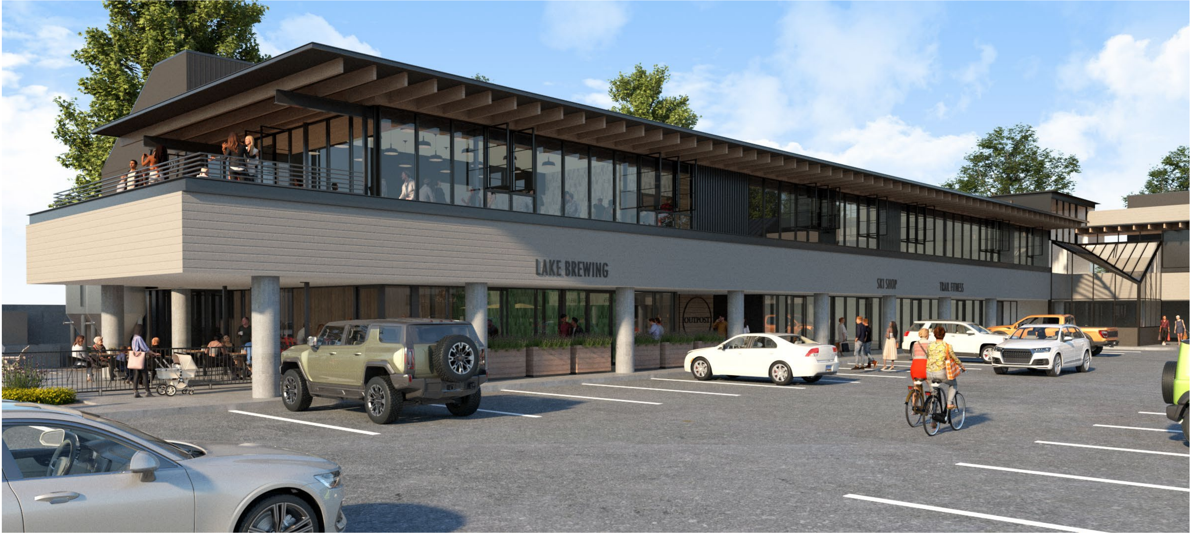
VIEW FROM ENTRY
