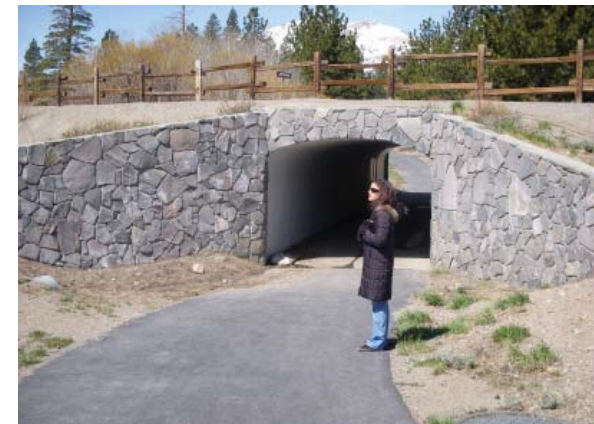
MAIN PATH UNDERPASS
