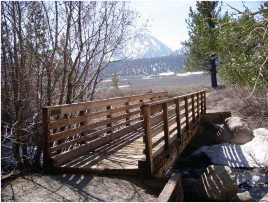
BRIDGE TO HAYDEN CABIN IN MAMMOTH CREEK PARK EAST
