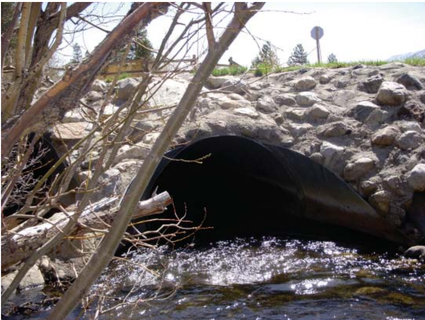
MAMMOTH CREEK IN CULVERT BELOW OLD MAMMOTH ROAD
