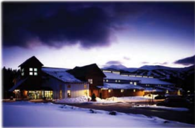
Indoor ice rink facility (Breckenridge, CO)
